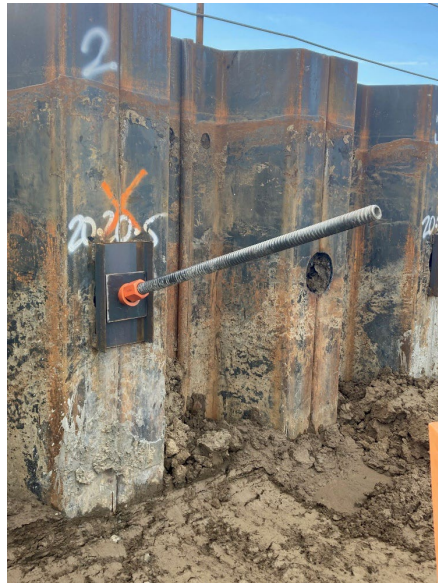
Sheet pile wall with tiebacks
